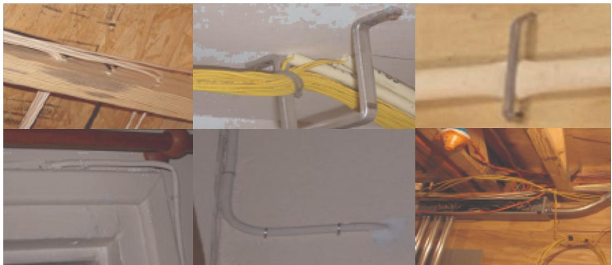
Figure 1. A montage of in-building installation and routing techniques that result in unusually tight bending for optical fiber.
